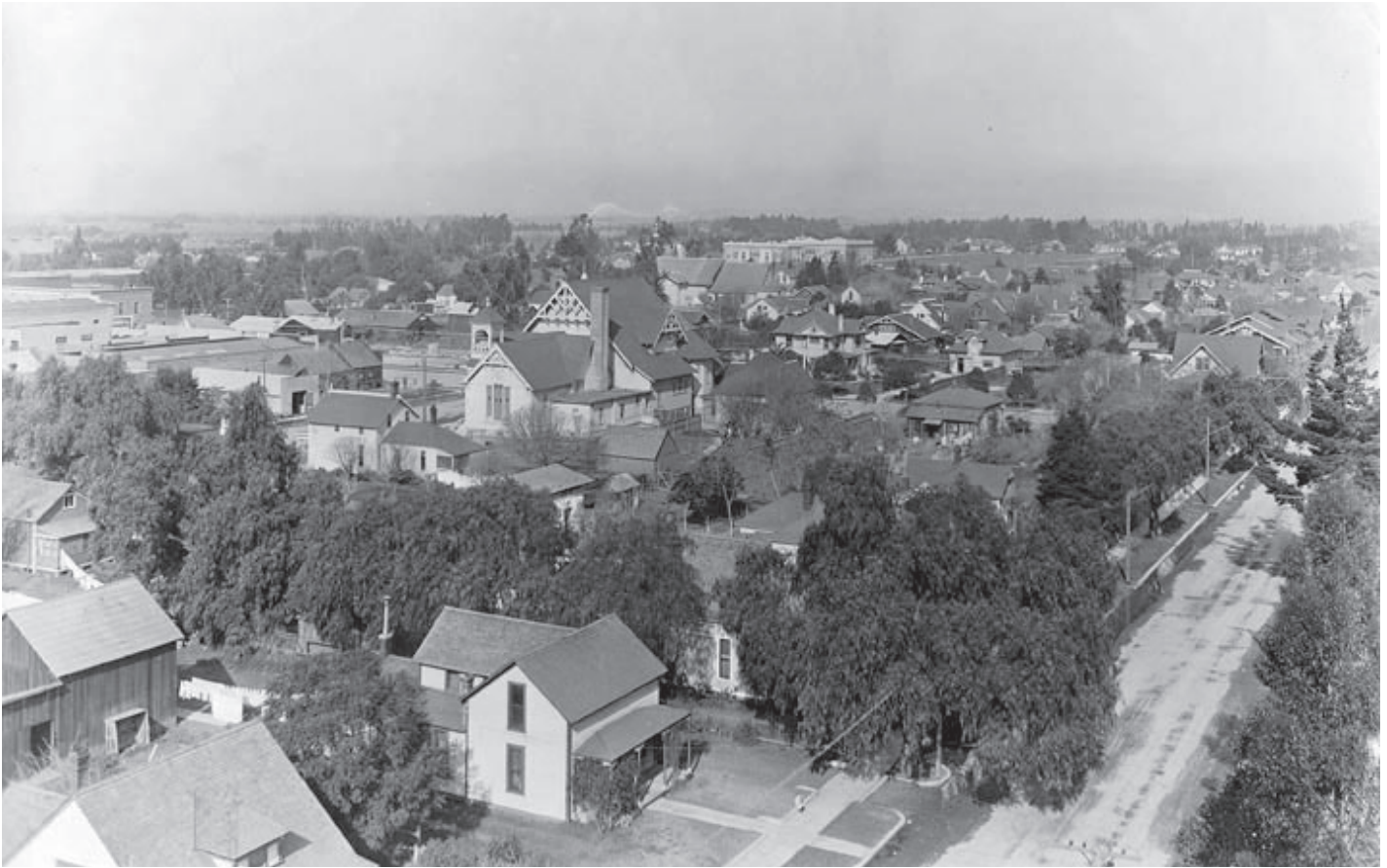
Figure 3. Orange, California, looking northwest from St. John's Lutheran Church, ca. 1914, Source: Orange Public Library and History Center
