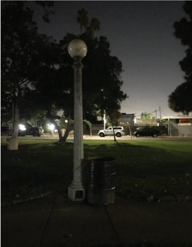
Figure 6. One of four lamp posts in the interior of the park. All four are either broken or non functional.
